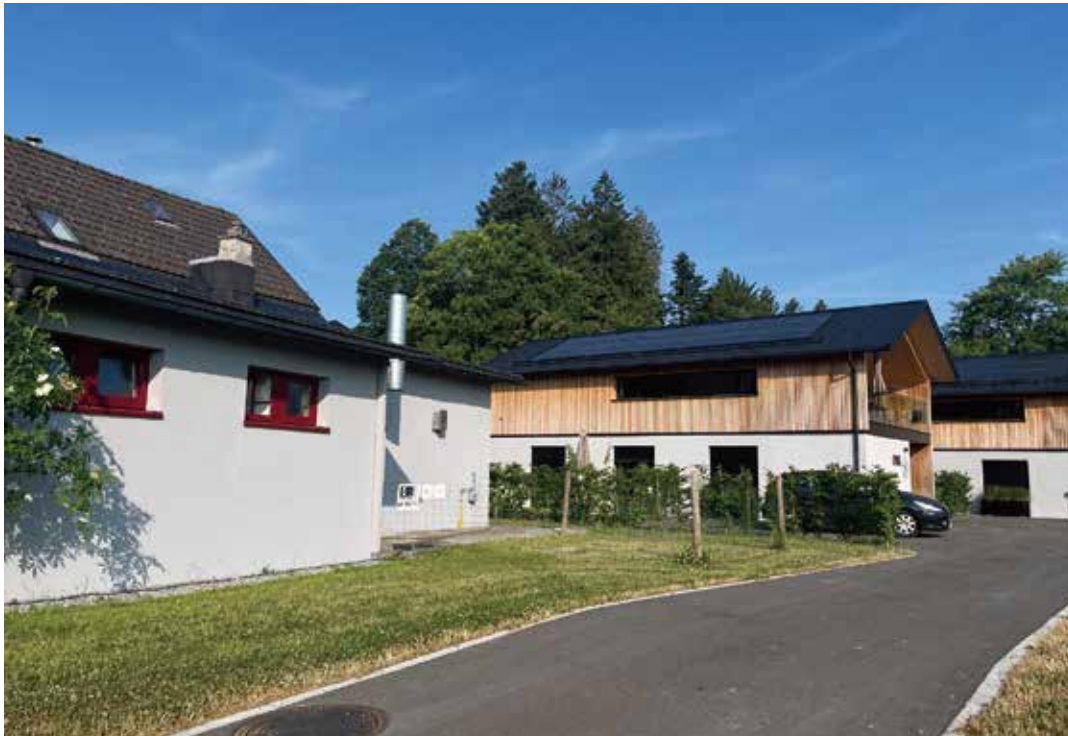
13 Residential ESS Project in Europe
