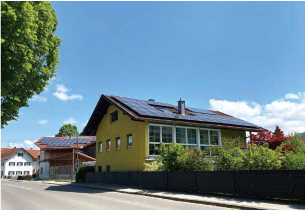
12 Residential ESS Project in Europe
