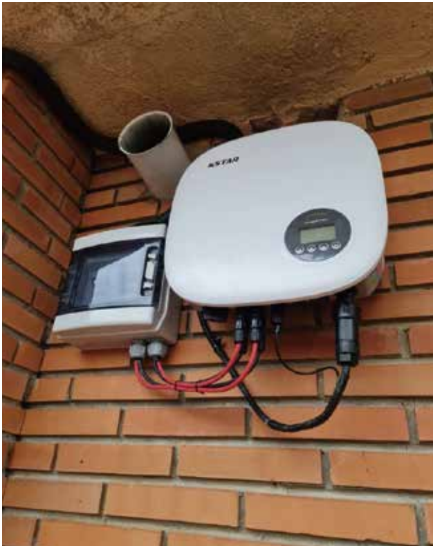
08 Residential Solar Project in Brazil
